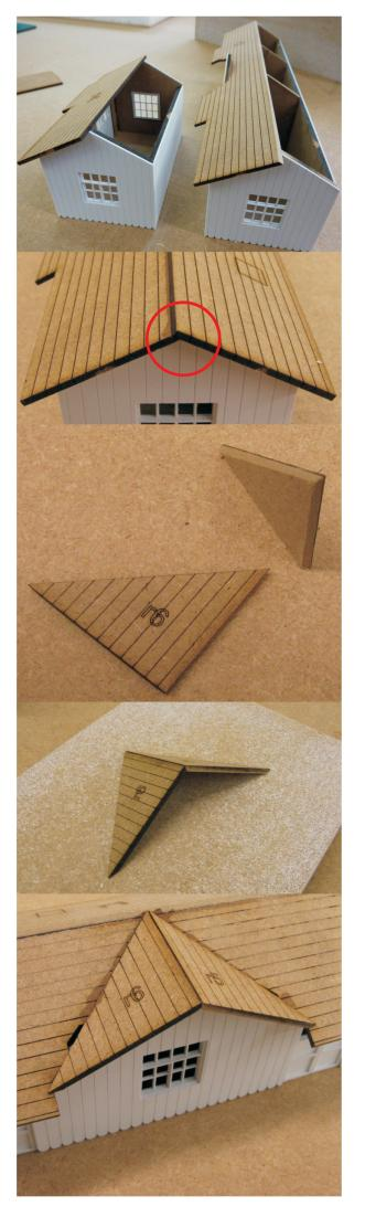
Next is the roof. You will need a large sanding block with approx 150-200 grit. Glue r2 on top of the structure as shown. Sand with a sanding block to follow the pitch of the roof on the other side then add r1 so it just overlaps r2 (see ) then sand it using a sanding block so it is flush with r2
